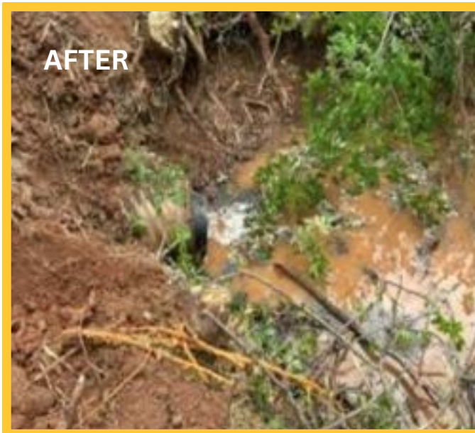
Slipline and Tail Pipe Dirt Work
