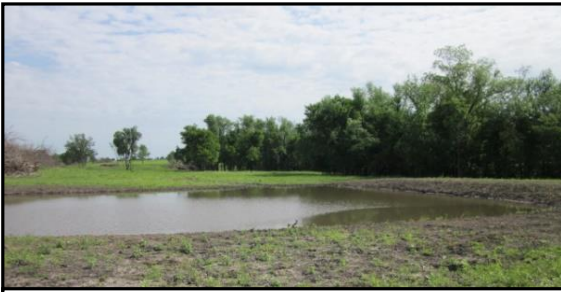
New Pond Construction
