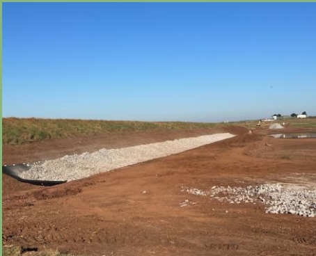
1,546 tons of riprap was required to protect 1,340 feet of front slope on Upper Black Bear watershed site 2 in Noble County.
