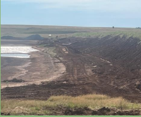
Lower Red Rock watershed 13 was drained and repaired due to front slope damage. 1,462 tons of riprap were used to protect 700 feet of slope.
