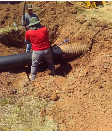
Tri-County Turkey Creek Watershed Site #11 getting repairs to Pipe Slip.
