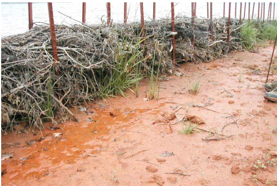
Fine sediment filled in the originally rocky shore following installation of the breakwater branch boxes. This sediment will support the establishment of dense vegetation to support shoreline stabilization.
