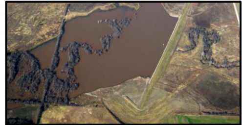
Upper Red Rock Creek Watershed Dam No. 52 protects I-35 and agricultural land
