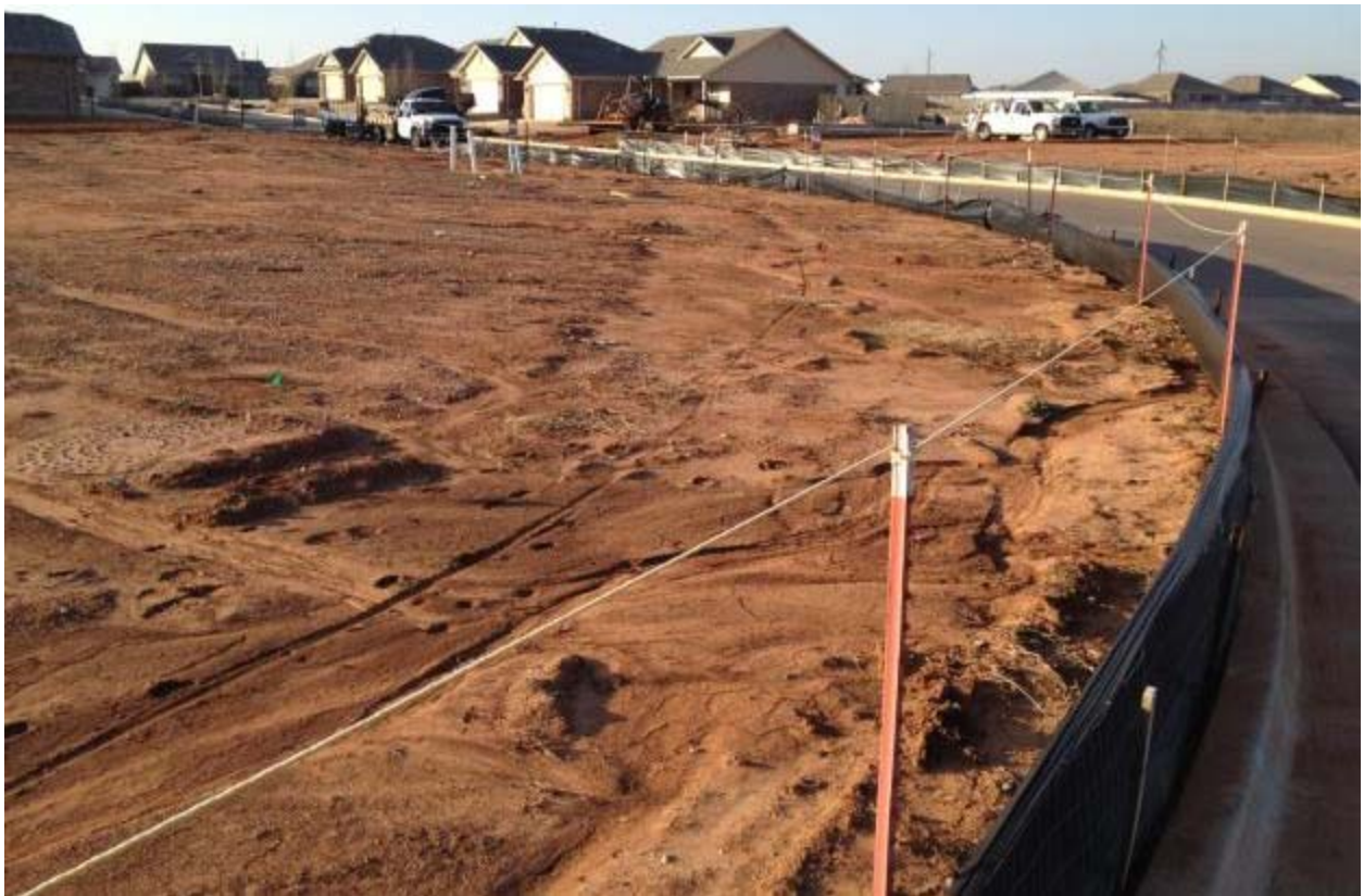
Figure 22: Photo of the rain gardens functioning as a mini sediment catch basin during construction.
