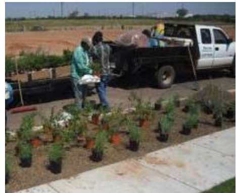
Figure 13: Shows the rain garden sub drain pipe installation with aggregate, fabric and sand (Top) and during parcel development as a mini catch basin (Bottom left), once completed the garden was excavated, filled with substrate (Bottom middle) and planted in the same day (Bottom right).
