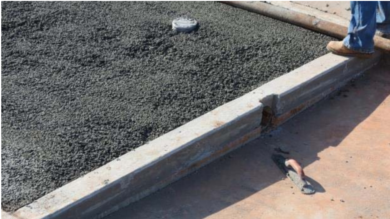
Figure 15: A small pad of porous concrete (120 s.f.) was placed over 36" of aggregate in the stormwater flume of the demonstration basin (Top). The pad accommodates both high flows to prevent flooding and the rain garden sub-drain pipe which daylights prior to the downstream test flume (Bottom). Wells were installed monitor sub-grade infiltration.
