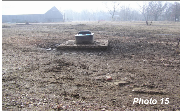
Freeze-proof water tank before and after geotextile and gravel protection.
