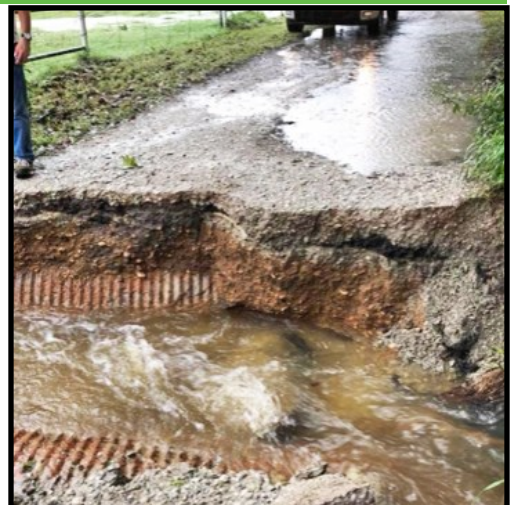
Road washed out in Pontotoc County due to heavy rains.
