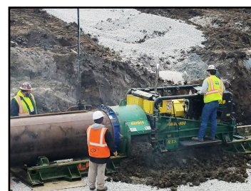
Steel Casing being bored and jacked into through an embankment.
