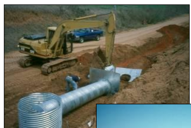
Grade stabilization structures divert water to prevent gully erosion and provide water for cattle.
