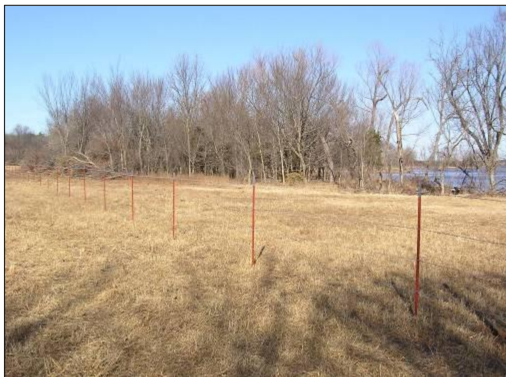
Riparian fencing similar to that above was installed for the Beaty Creek project and the Sandy and Yellowstone Creek projects. Fencing excludes cattle from the stream and banks, allowing vegetation to both stabilize the banks and filter rain and irrigation runoff from croplands and pasturelands.
