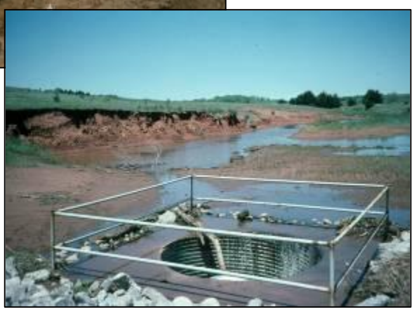
Grade stabilization structures divert water to prevent gully erosion and provide water for cattle.
