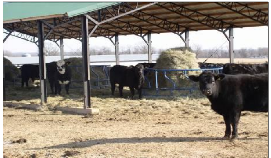
A winter feeding facility for cattle was a BMP installed for this project. These facilities are sited to help concentrate animal waste away from streams.
