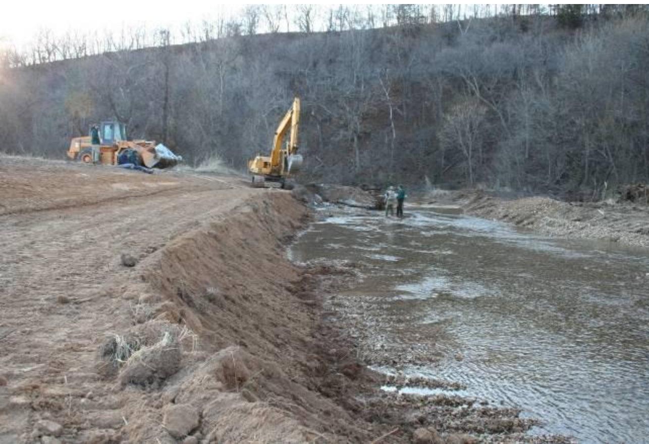
Channel stabilization project at Honey Creek in northeastern Oklahoma
