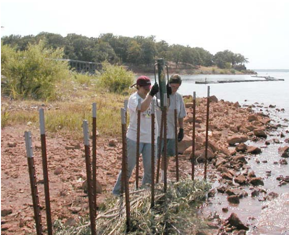
Figure 10: Left – Driving t-posts. Right – Packing branch wattles.
