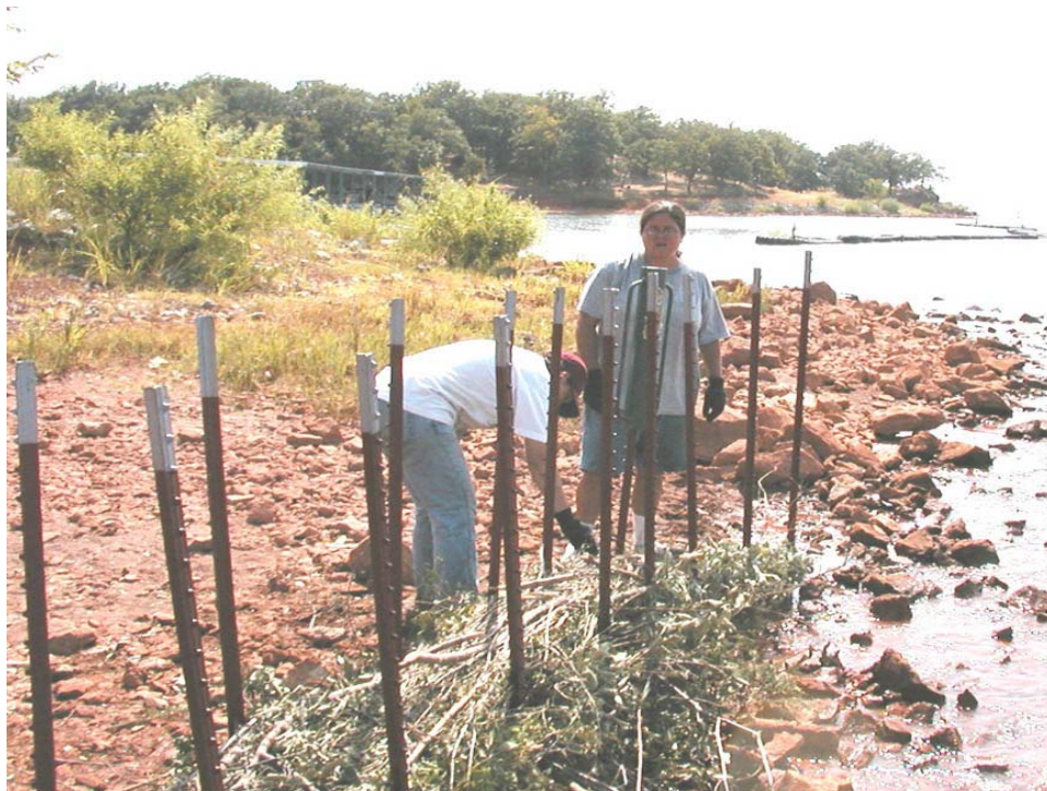
Figure 9: Installing “wattles” (branch bundles) into branchbox.
