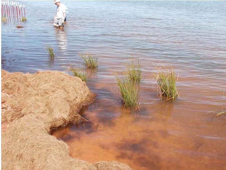
Figure 20: July 14, 2004 - Assessment of CGR breakwater collapse after storm event. Coconut fiber rests on the shore with remaining plants once protected by the CGR.
