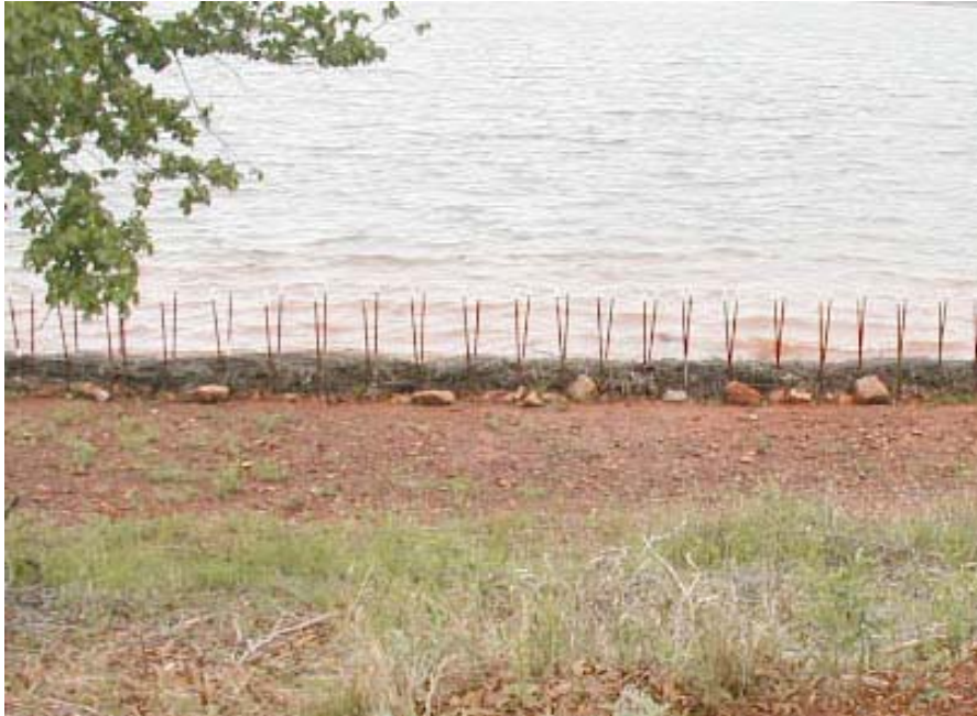
Figure 11: Completed branchbox (1.5 ft. below conservation pool).
