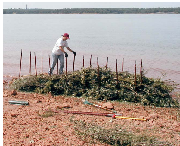
Figure 10: Left – Driving t-posts. Right – Packing branch wattles.
