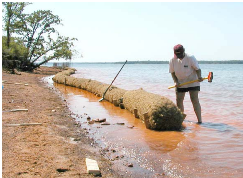
Figure 12: Staking a CGR.
