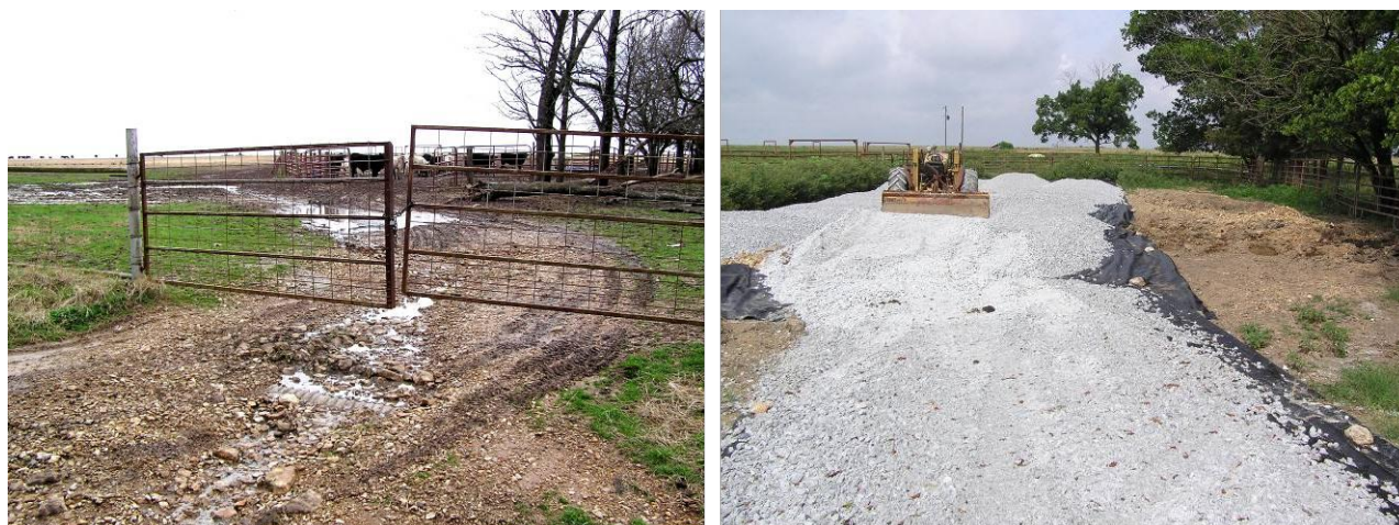
Figure 21. Installation of Heavy Use Area Protection in the Beaty Creek Watershed to Reduce Runoff of Nutrients, Sediment, and Bacteria.
