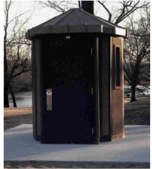
Figure 3. Prefabricated permanent pit toilet facilities installed at Round Hollow Public Access Area along the Illinois River.
