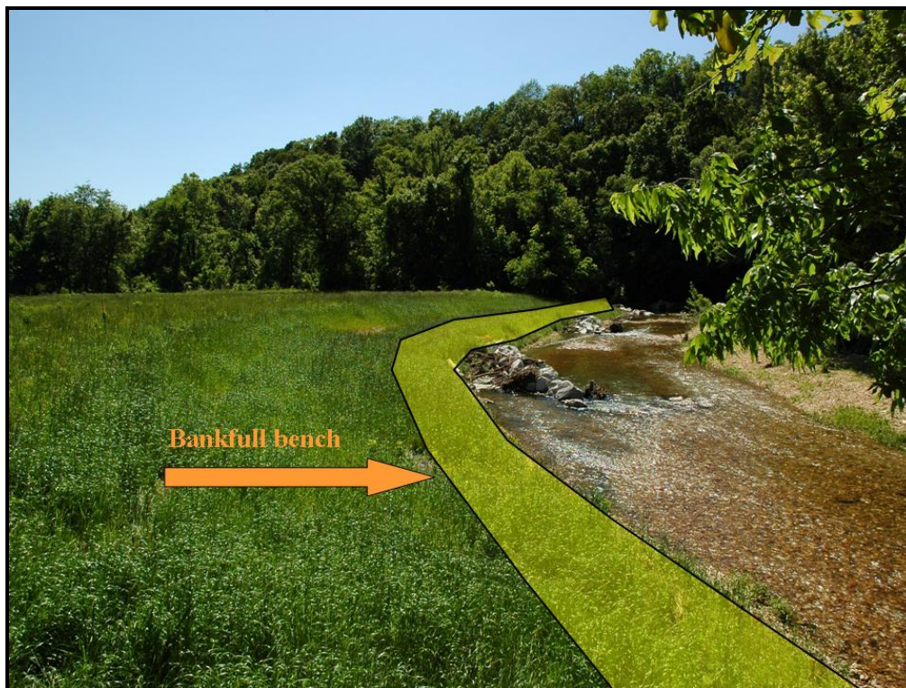
Figure 5: Constructed and vegetated bankfull bench
