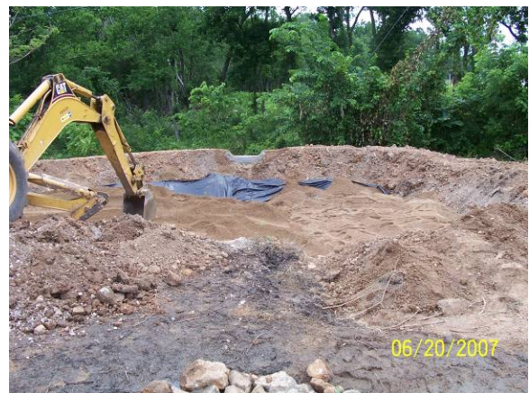
Top Left: Site prior to cell construction. Middle Left: Drainage pipe layout. Bottom left: Load of mixed filter medium ready to be placed in cell. Top Right: Completed drainage. Middle Right: View of liner used to stabilize cell wall. Bottom Right: Installation of one lift of filter layer.
