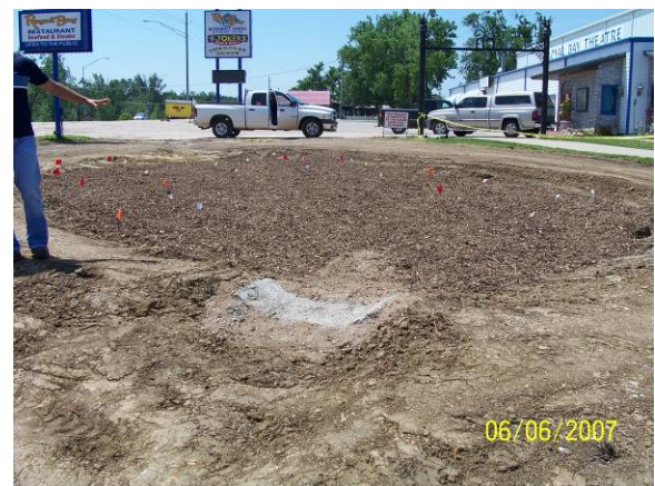
Top Left: Partially backfilled cell. Middle Left: Flags marking sand plug locations. Bottom left: Completed top soil / sand plug layer. Top Right: Application of hardwood mulch. Middle Right: Completed, unplanted cell. Bottom Right: Overflow weir.
