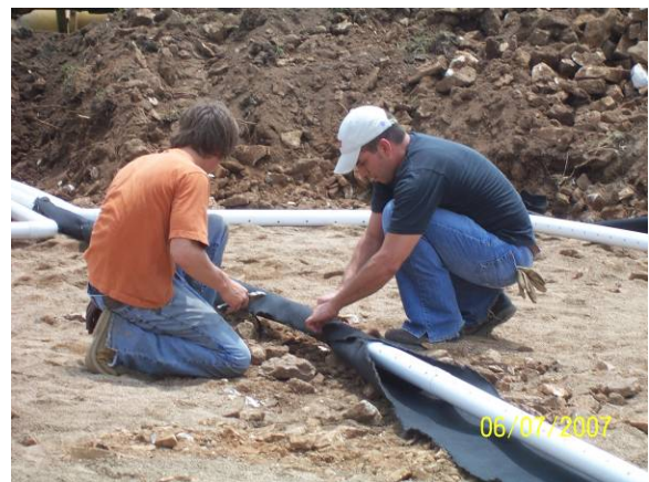
Top Left: Site prior to cell construction. Middle Left: View of rocky soil conditions encountered during excavation of this site. Bottom left: Cell excavation. Top Right: Application of sand lift prior to drainage pipe placement due to rocky site conditions. Middle Right: Drainage pipe placement. Bottom Right: Securing filter fabric to drainage pipe.
