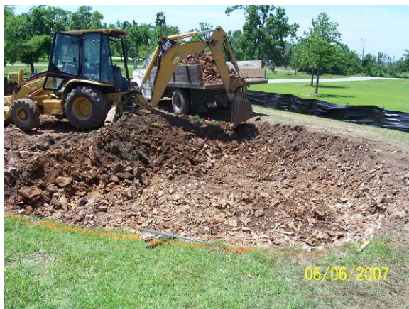
Top Left: Site prior to cell construction. Middle Left: View of rocky soil conditions encountered during excavation of this site. Bottom left: Cell excavation. Top Right: Application of sand lift prior to drainage pipe placement due to rocky site conditions. Middle Right: Drainage pipe placement. Bottom Right: Securing filter fabric to drainage pipe.
