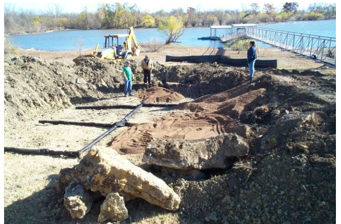
Top Left: Site prior to cell construction. Middle Left: View of cell boundaries. Bottom left: Drainage outlet installation. Top Right: Cell excavation. Middle Right: Installation of drainage system. Bottom Right: Placement of filter layer lift.
