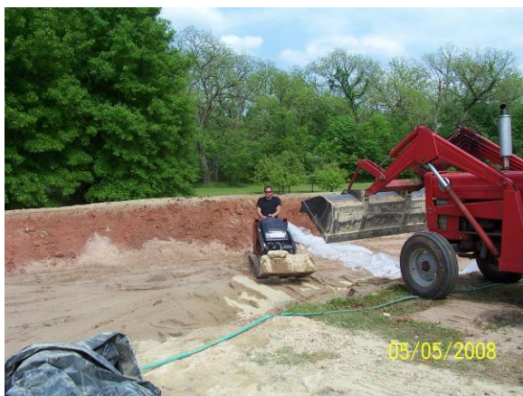
Top Left: Dingo leveling sand lift. Middle Left: Adding fly ash to sand. Bottom left: Dingo spreading fly ash evenly over sand lift. Top Right: Spreading fly ash over sand lift. Middle Right: Tilling fly ash into sand lift. Bottom Right: Completed filter layer.
