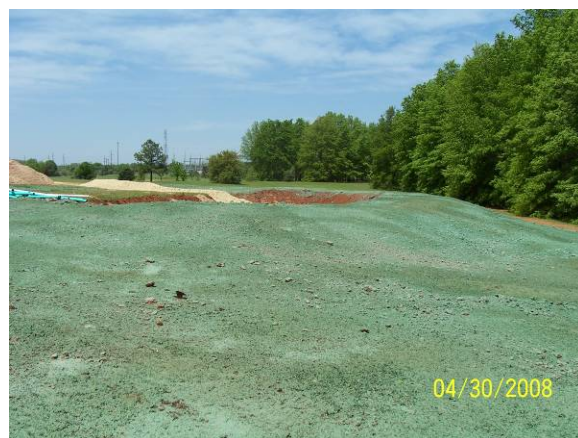
Top Left: Excavation of Cell B. Middle Left: Construction of berms for Cell B. Bottom left: Excavation of Cell A. Top Right: Excavation of drainage outlet for Cell B. Middle Right: Hydromulching cell berms. Bottom Right: View of hydromulched berm for Cell B.
