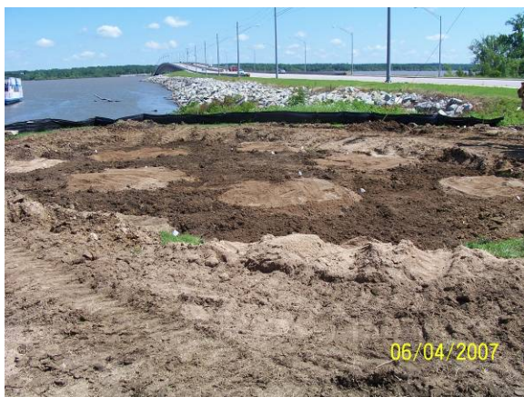
Top Left: Partially backfilled cell. Middle Left: Flags marking sand plug locations. Bottom left: Completed top soil / sand plug layer. Top Right: Application of hardwood mulch. Middle Right: Completed, unplanted cell. Bottom Right: Overflow weir.
