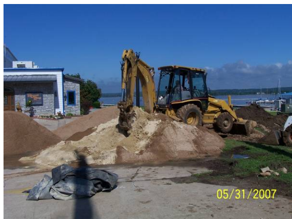
Top Left: Site prior to cell construction. Middle Left: Adding fly ash to sand. Bottom left: Mixing fly ash and sand for filter layer. Top Right: Completed drainage. Middle Right: Alternate view of drainage. Bottom Right: Front end loader backfilling filter media.
