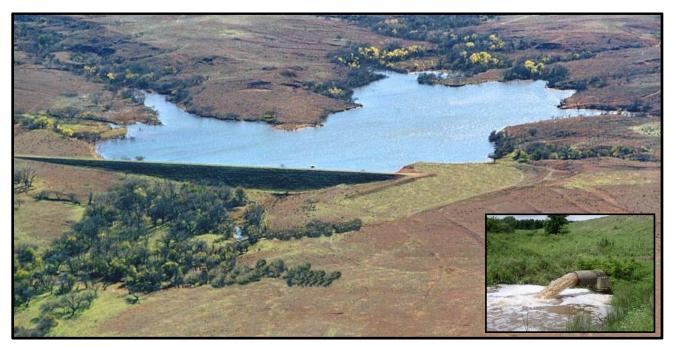
Flood control dams impound water during heavy rainstorms and slowly release it through a pipe through the dam over a period of several days or weeks. This reduces the amount of rainwater that reaches a stream or river immediately after a storm and reduces flooding.
