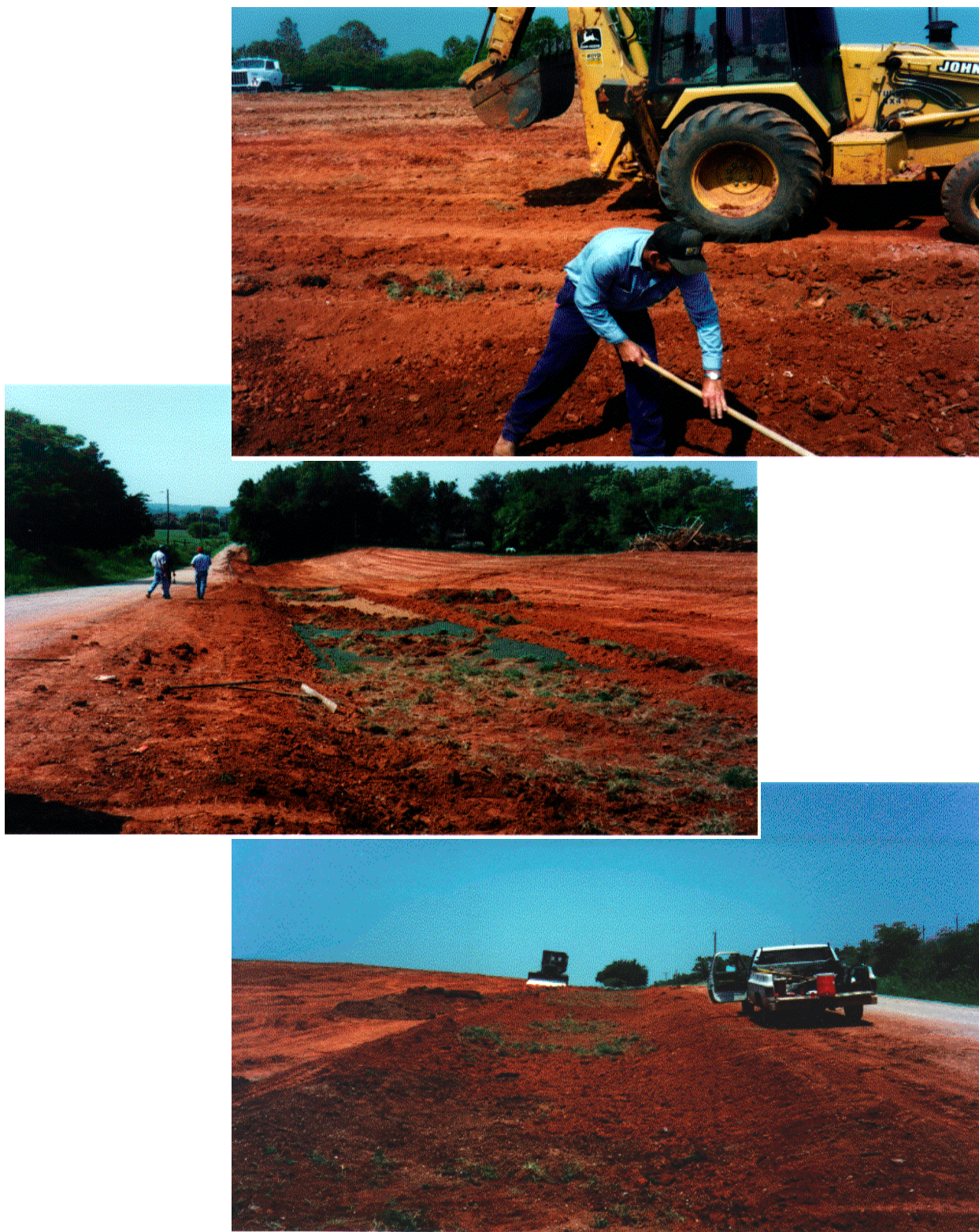
Figure 3.9 Soil Cover Placed Over Erosion Control Blankets.
