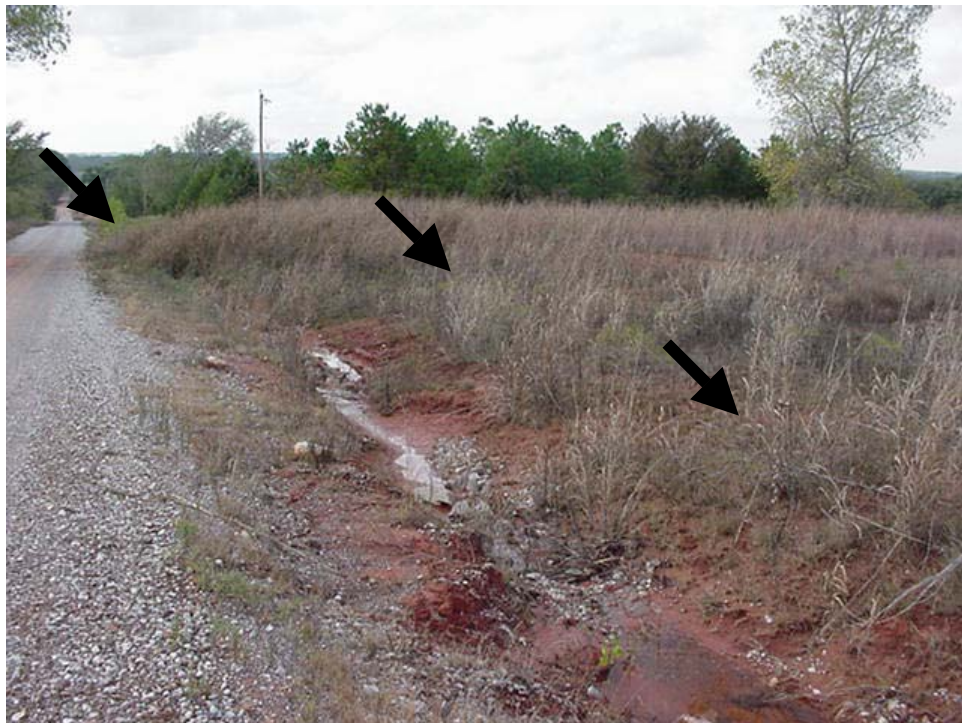
Figure 4.23 Site 2 Looking West About 1.5 Years After Erosion Control (Fall 2000). [Note vegetation (arrows) in vicinity of telephone pole and along road not observed in Fig. 4.22]
