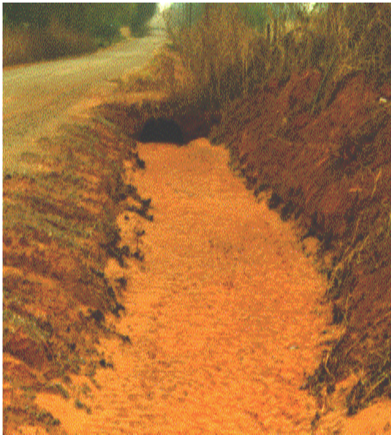
Figure 1.2 Sediment Deposition in a Culvert Along a County Road due to Upstream Erosion (location is south of Site 1).
