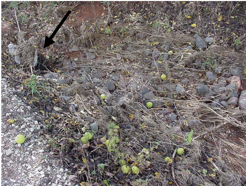
Figure 3.7 Rock Placed to Protect Soil Near Culvert Entrance. [Arrow points to culvert]
