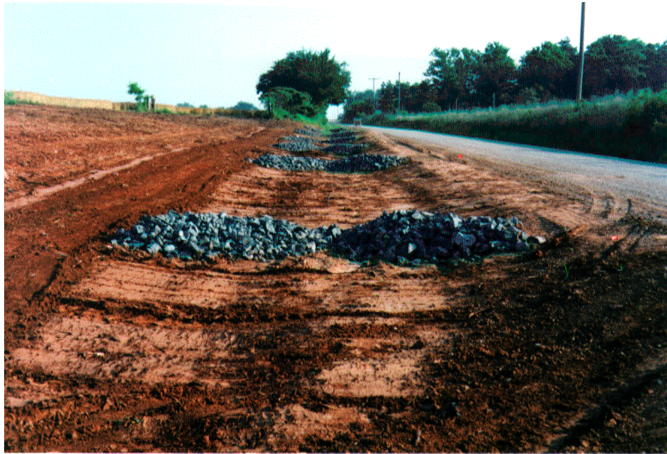
Figure 3.6 Rock Berms Placed at Site 1.
