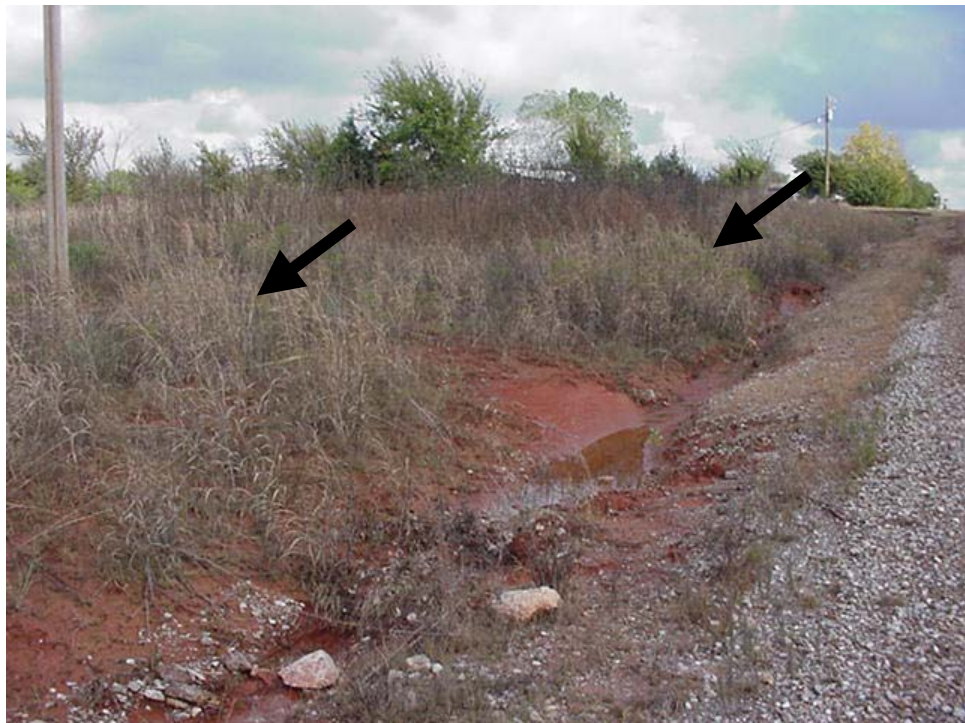
Figure 4.21 Site 2 Looking East About 1.5 Years After Erosion Control (Fall 2000). [Note vegetation (arrows) in vicinity of telephone pole and along road not observed in Fig. 4.20]
