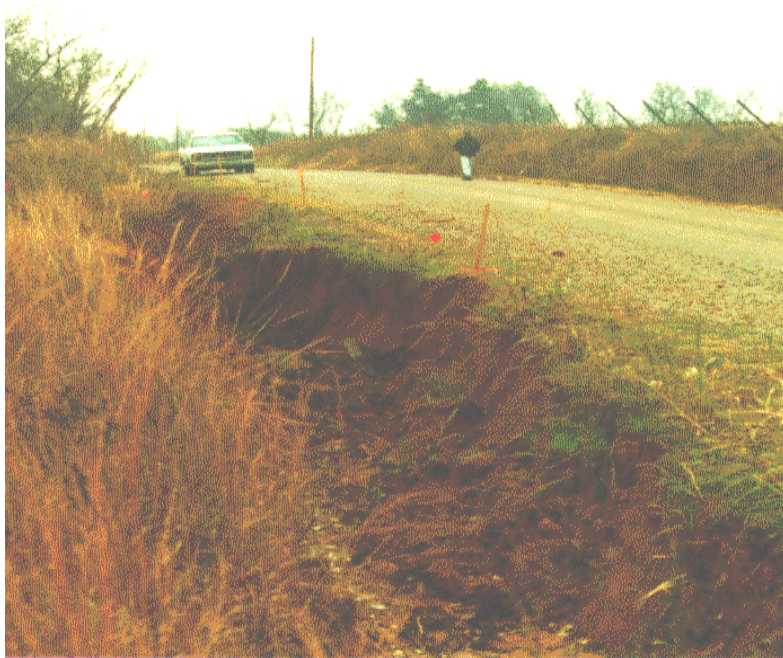
Figure 1.1 Severe Erosion Damage Along the Shoulder of a County Road (looking north at Site 1).
