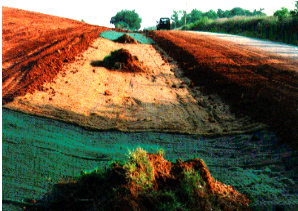
Figure 3.8 Erosion Control Blankets at Site 1.
