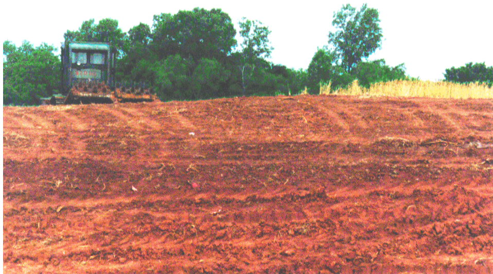
Figure 3.2 Compaction at Site 1 with Bulldozer and Sheepfoot Roller.
