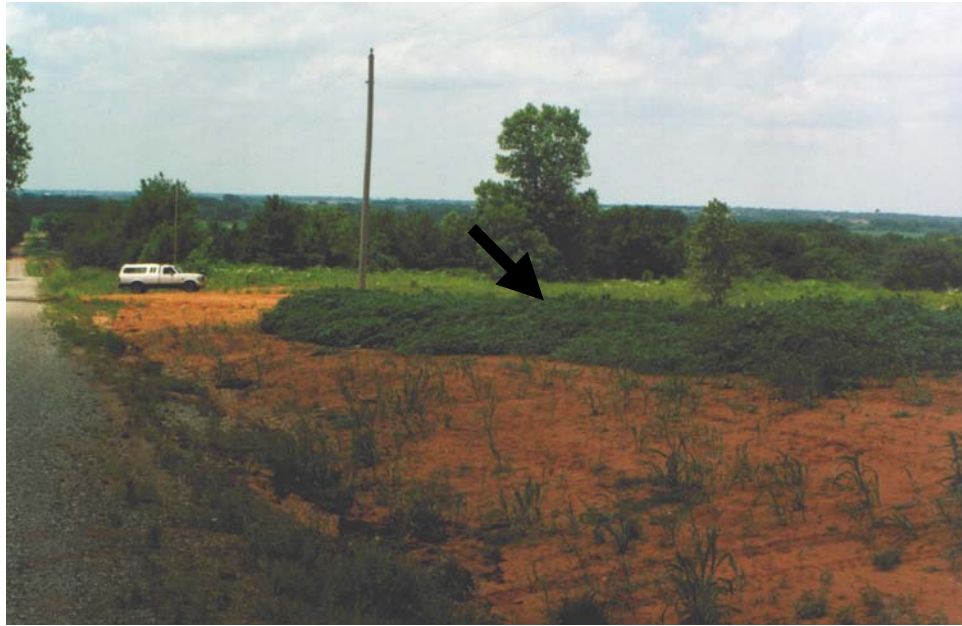
Figure 4.22 Site 2 Looking West 1.5 Months After Erosion Control (Spring 1999). [Note area of thick vegetation (arrow) where cotton burrs were placed.]
