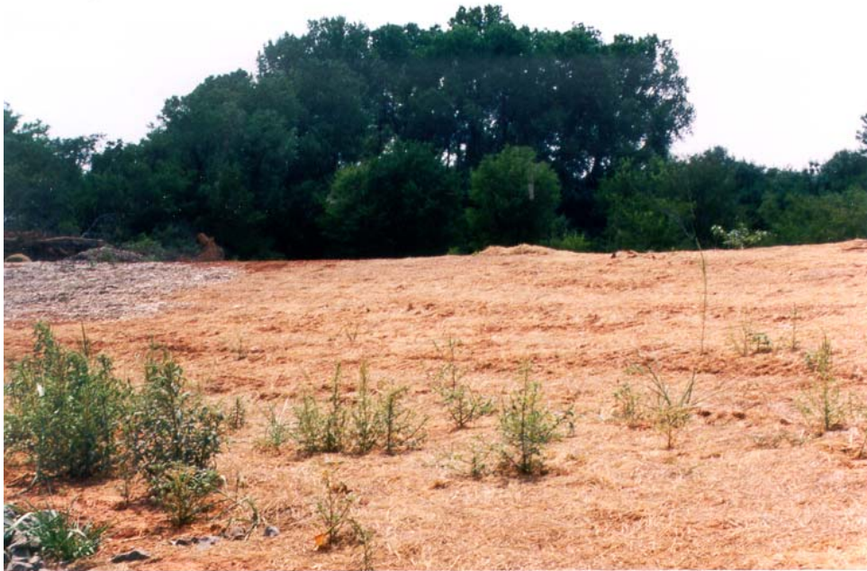
Figure 3.4 Hay Mulch at Site 1 with Limited Vegetation.
