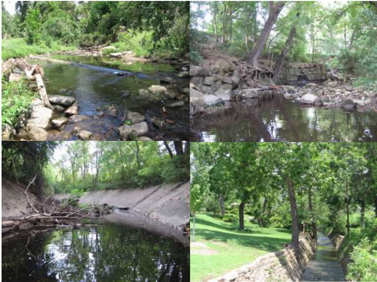
Figure 5: Sanitary sewer main in creek (top left) and examples of riprap (top right) and channelization (bottom) along Crow Creek in Tulsa County, Oklahoma.
