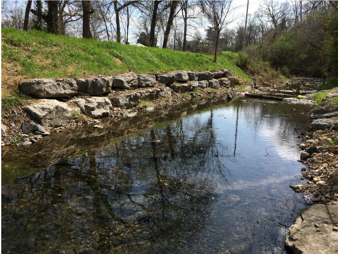
Figure 18. History Trail from right bank looking downstream depicts the left bank boulder placement utilized to stabilize the bank toe.
