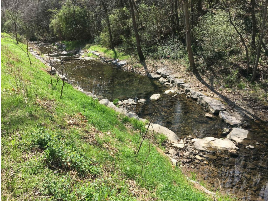
Figure 17. History Trail in Spring 2017 left bank looking downstream. The bench has been reconstructed, anchored with boulders, and replanted with trees and grasses.
