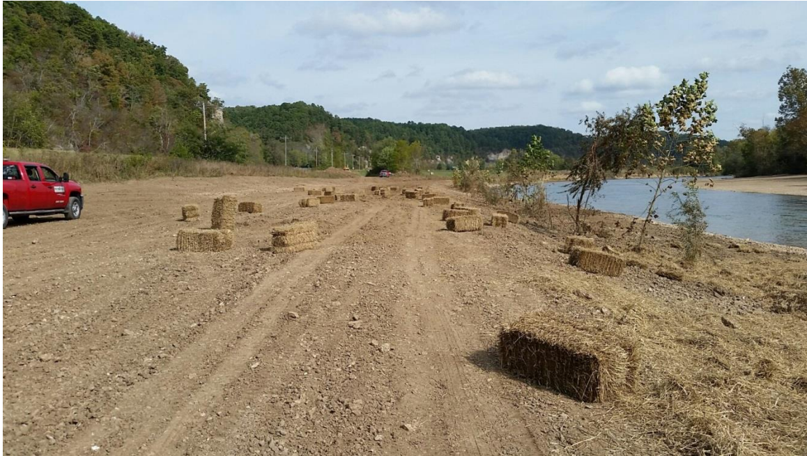
Figure 8. Preliminary mulching and seeding occurred in late October, although full planting was planned for December. Trees were transplanted from the opposite bank and rootballs placed near the water level to promote optimal survivability.
