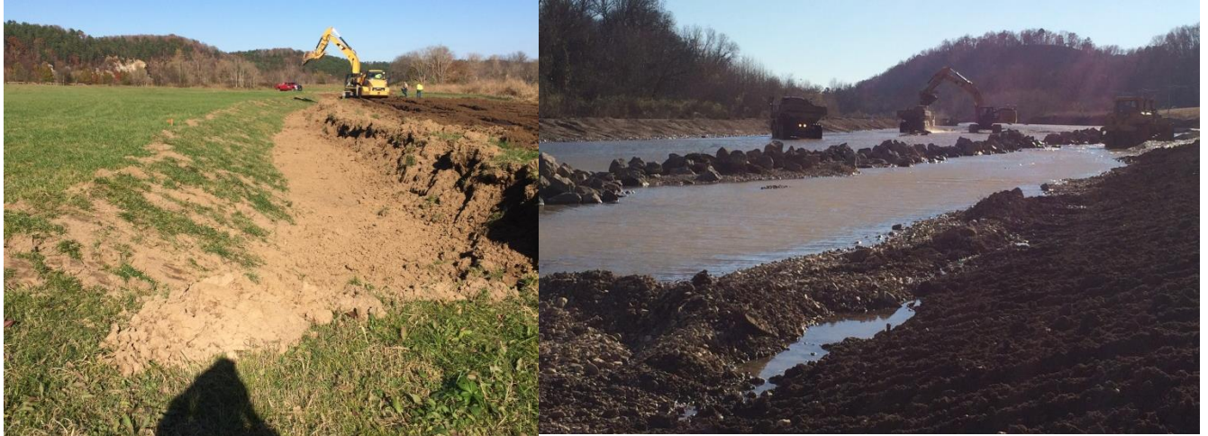
Figure 4. Construction of Bankfull Bench and Channel Reconfiguration begun in Fall 2015.
