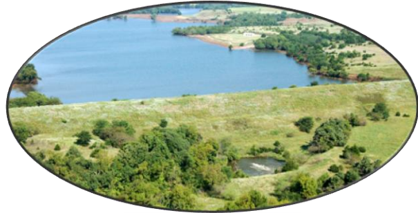
Cobb Creek Dam No. 1 before rehabilitation
