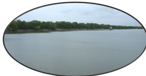
Caddo Creek Watershed Dam No. 13 (Lake Jean Neustadt) provides flood control and municipal water for the City of Ardmore.
