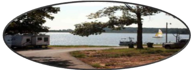
Big Wewoka Creek Watershed Dam No. 22 provides flood control and recreational areas.
