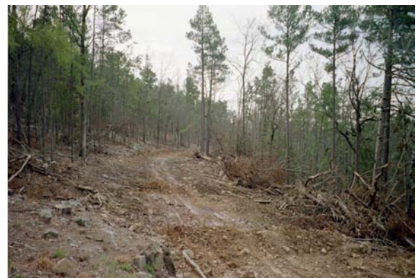
Properly installed waterbars on a mountain haul road in eastern Oklahoma.
