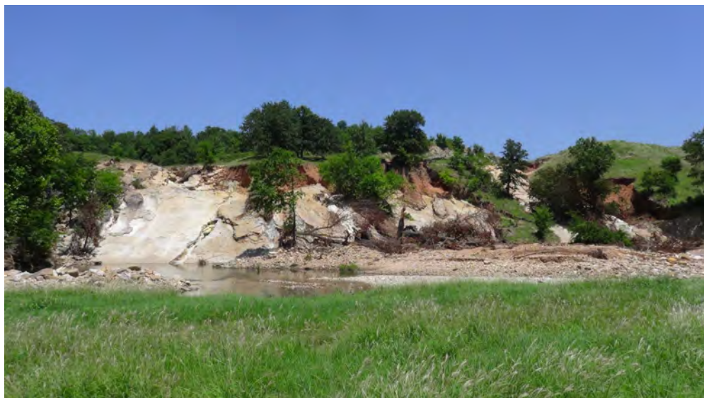
Severe damage to the auxiliary spillway of Caddo Creek Site 27, June 2015.
