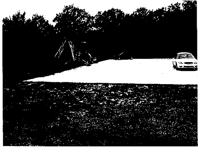
Earthwork begins on a new rain garden at Remington Elementary in Tulsa. The Oklahoma Conservation Commission and the City of Tulsa are partners with the Indian Nation Council of Governments. Local volunteers will help with planting and the laying of sod.
