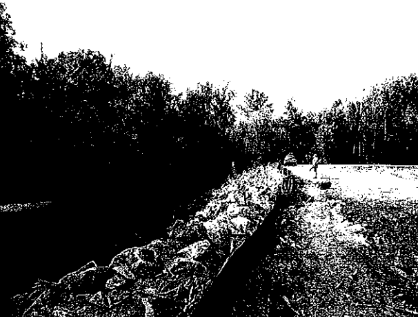
Left: Documentation of road work at the Spring Creek ( Mayes County ) Blue Thumb site. NOTE: Silt fence is adequately installed.
