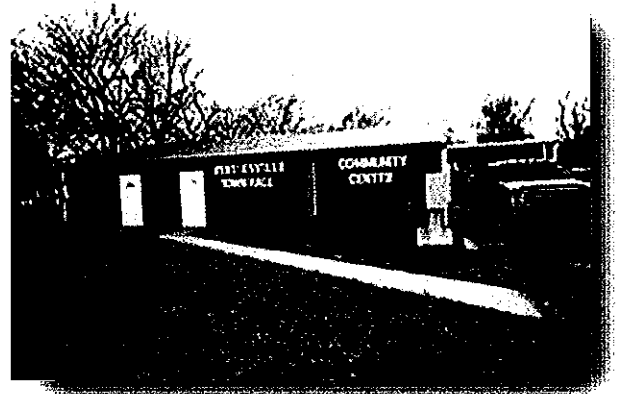
Rentiesville, OK Town Hall and Community center on Tuesday, April 7, 2015. This facility will be replaced by a new community center funded with assistance of the U.S. Department of Agriculture (USDA), rural Development (RD)
