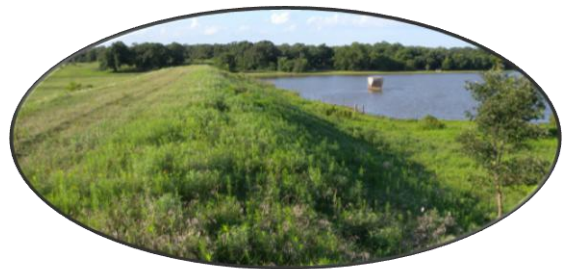
Five of the 107 flood control dams also provide municipal water and recreational areas.
