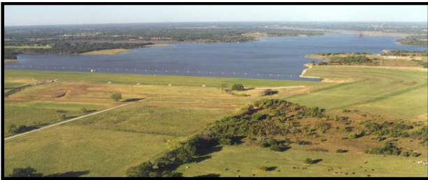
North Deer Creek Dam No. 1 in Pottawatomie County is one of the dams that was constructed for flood control, municipal water supply and recreational areas.
