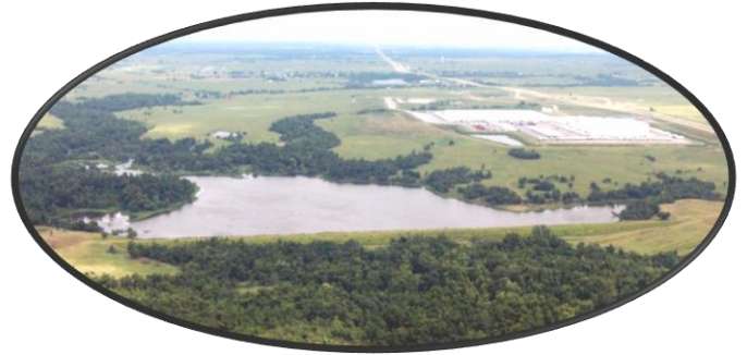
Double Creek Watershed Dam No.1 after it was rehabilitated.
