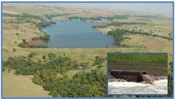
Flood control dams impound water from high rainfall events and release it slowly over a period of days or weeks. This reduces flooding downstream.
