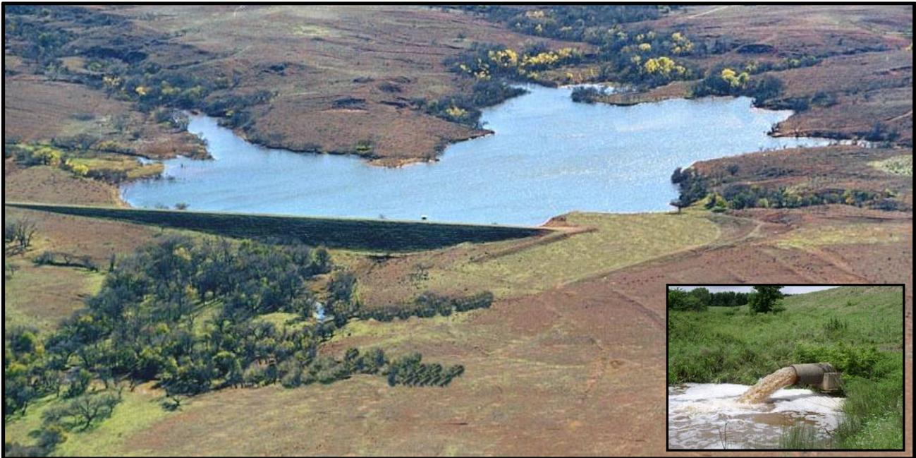
Flood control dams impound water during heavy rainstorms and slowly release it through a pipe through the dam over a period of several days or weeks. This reduces the amount of rainwater that reaches a stream or river immediately after a storm and reduces flooding.
